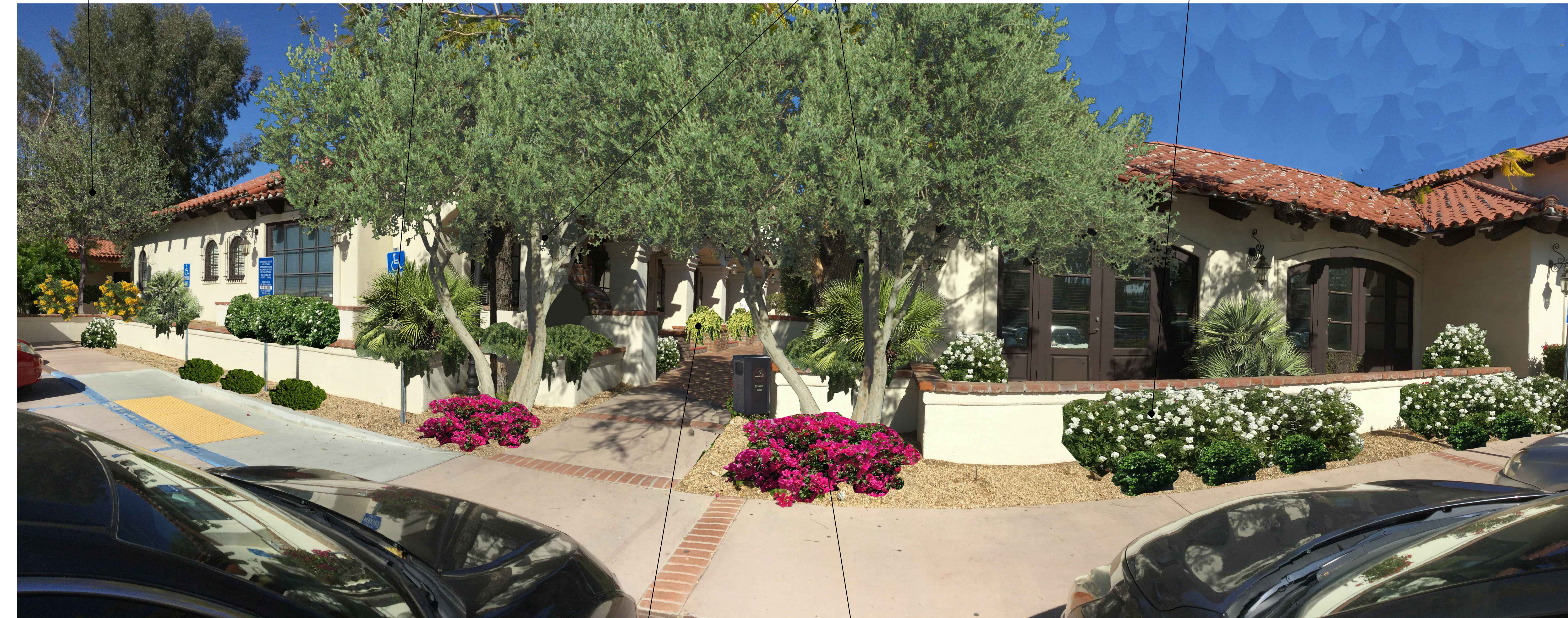
AFTER WEST COURTYARD ACCESS
