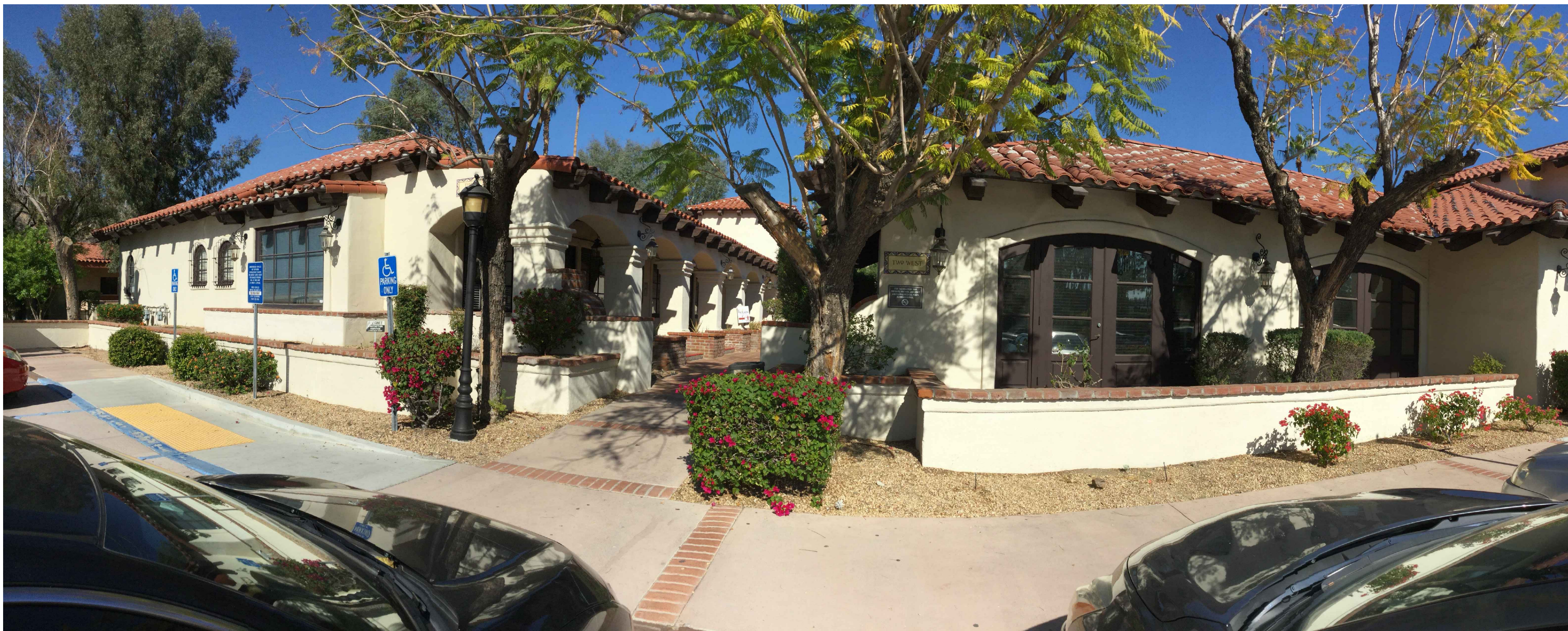
BEFORE WEST COURTYARD ACCESS
