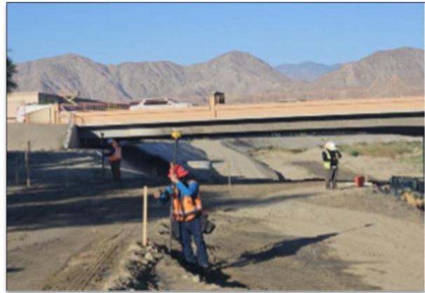
Grading at Jefferson UC.
