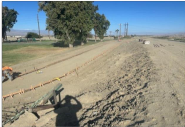
Formwork install at Sierra Vista Park Connector in Coachella
