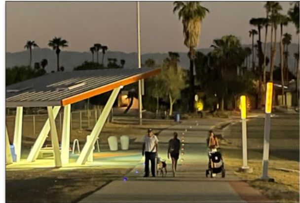
Light columns are installed at the Demuth Park Access Point in Palm Springs.
