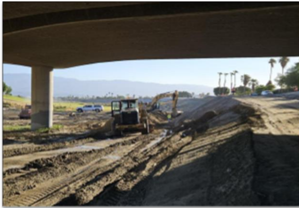
Grading continued at Jefferson UC.
