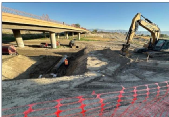
RCP extension and compaction at Jefferson UC.
