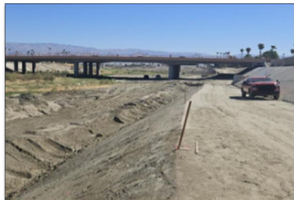
Grading of CSP at Jefferson UC (west).
