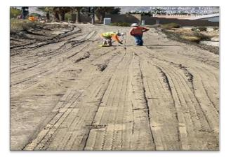
Importing, placing, grading, and compacting subgrade for placement of JPCP; Sunrise Way to Gene Autry in Palm Springs.
