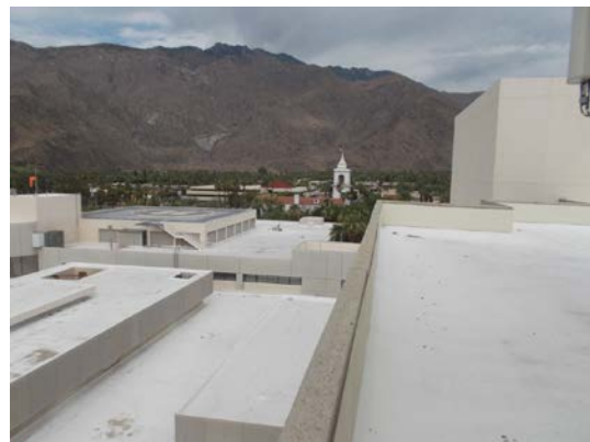
VIEW OF ROOF WITH MOUNTAINS IN THE DISTANCE
