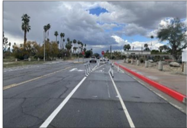
Delineators and striping upgrades added to the bike lane entrance of CV Link at El Cielo and Mesquite.
