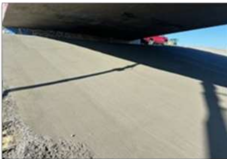
Avenue 52 undercrossing slope protection in Coachella.
