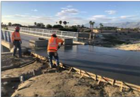
La Quinta path bridge connection (west).
