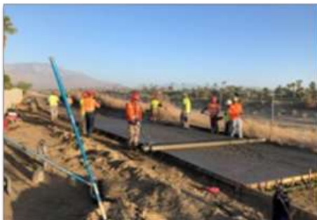
Concrete placement adjacent to Deep Canyon Dr. in Palm Desert.
