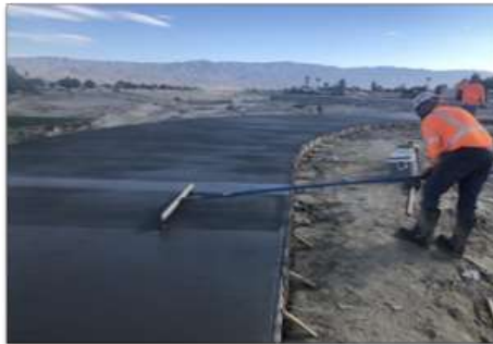
La Quinta path bridge connection (west).
