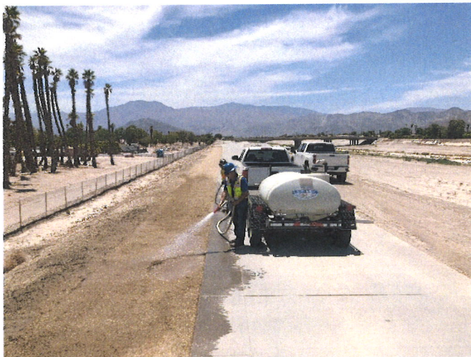
Continued DG install from Fred Waring to Indio Blvd
