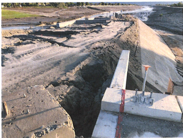
LQ Promontory Point subgrading damage from tropical storm.
