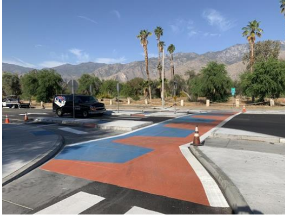
El Cielo and Mesquite Crosswalk Stripping
