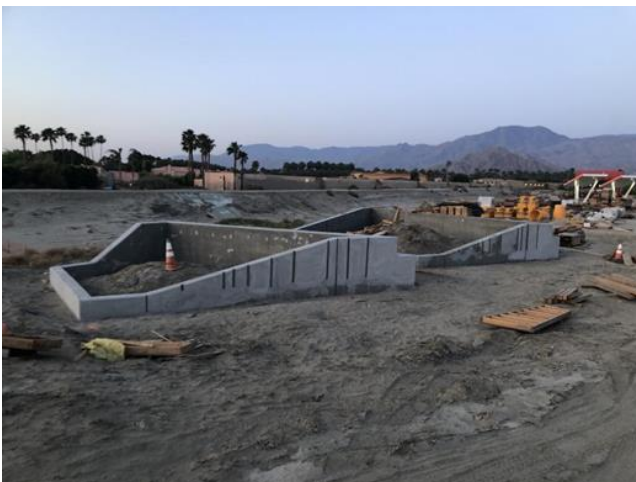
Finished Stadium Seating Walls Promontory Point
