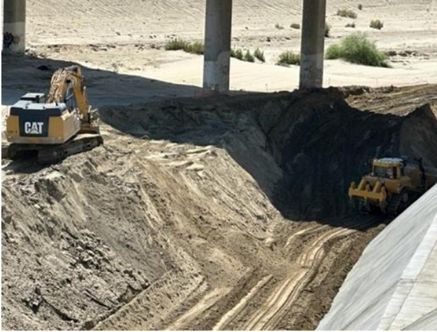
Cut off wall backfill operation at Golf Center Parkway
