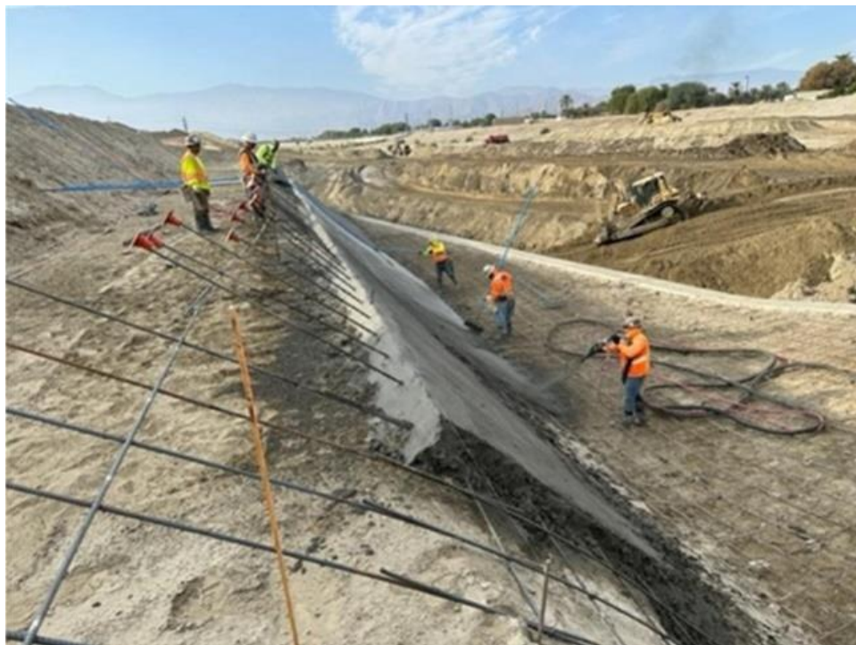
Photos of Pouring Adams Street Connector and Fred Waring Slope Protection.
